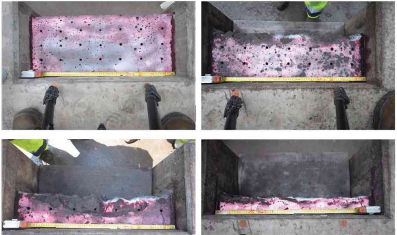
Figure 134: Crack detection on top Block B01 (Reference)
