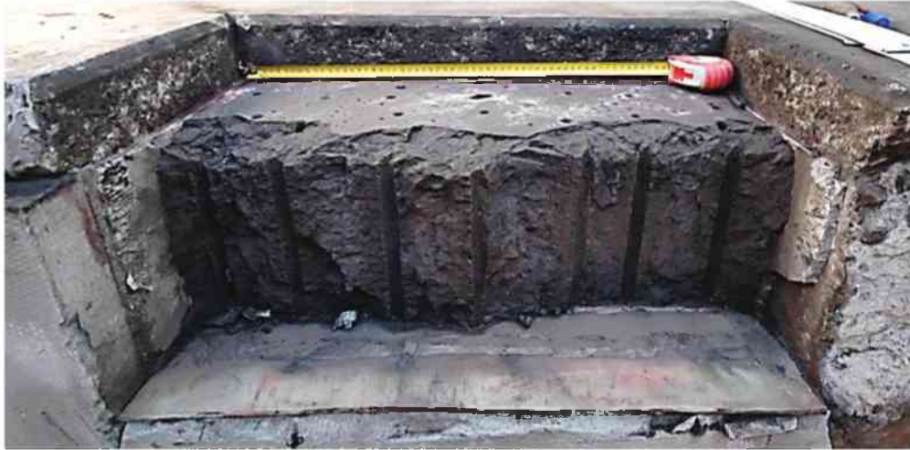
Figure 62: Front view after blasting of S+B variations pattern B04 row 1
