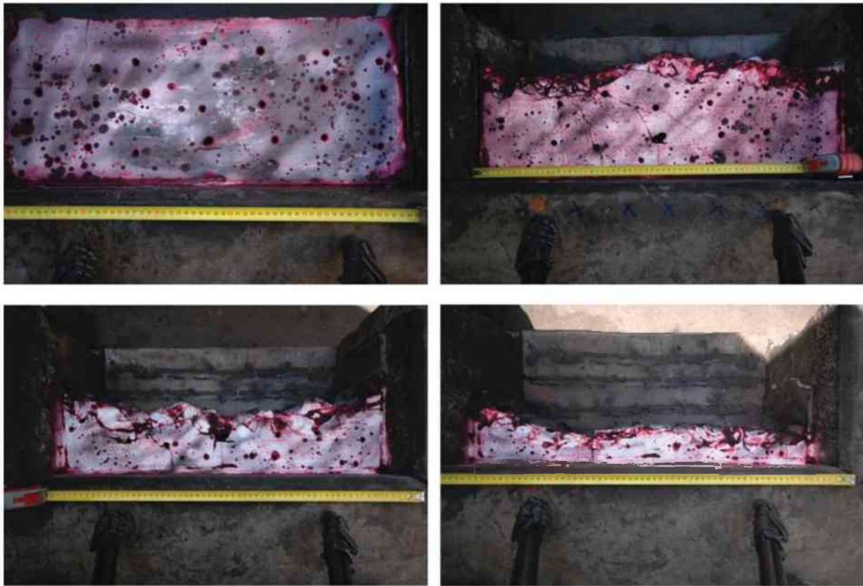
Figure 138: Crack detection on top Block B04 (S+B variations)
