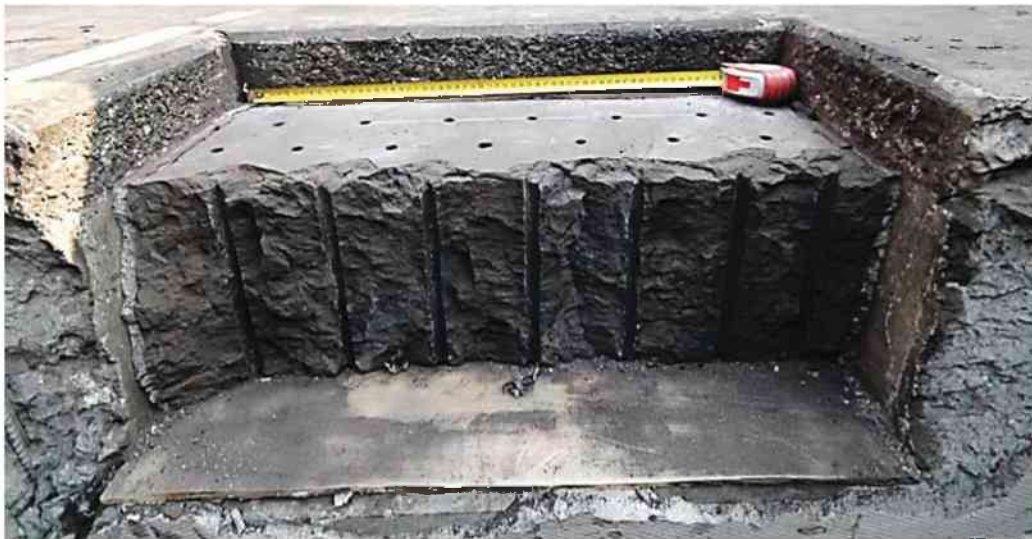
Figure 63: Front view after blasting of S/4 shift pattern B07 row 1
