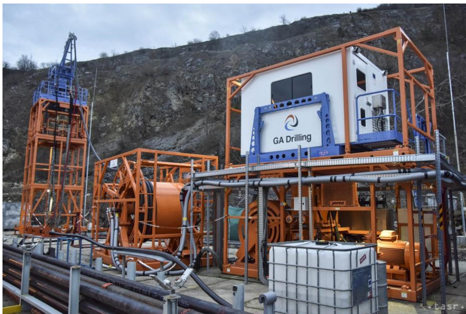
Figure 8 Pulsed plasma drilling surface facility (TASR, 2018)
