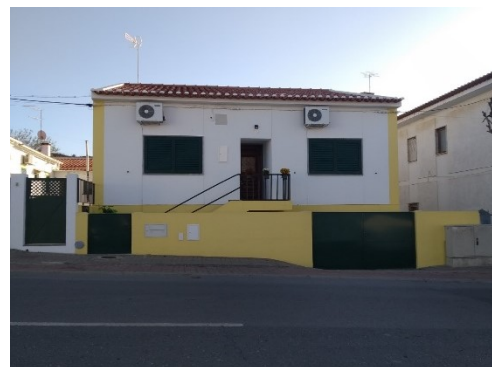
Figure 29 - Structure F: residential building.
