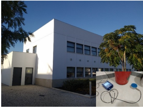
Figure 24 - Structure C: Aljustrel Town Hall.
