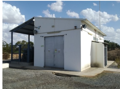
Figure 33 - Structure J: primary ventilation fan ancillary facility.
