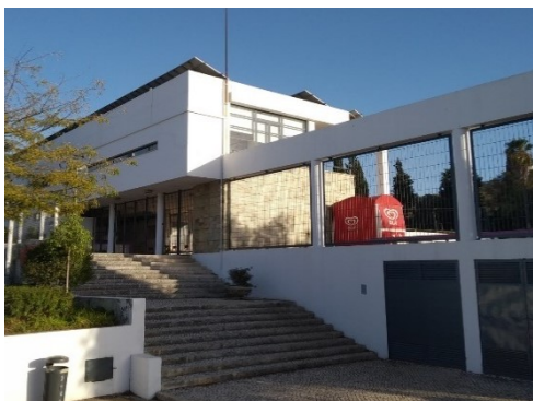
Figure 28 - Structure D: swimming pool ancillary facilities.
