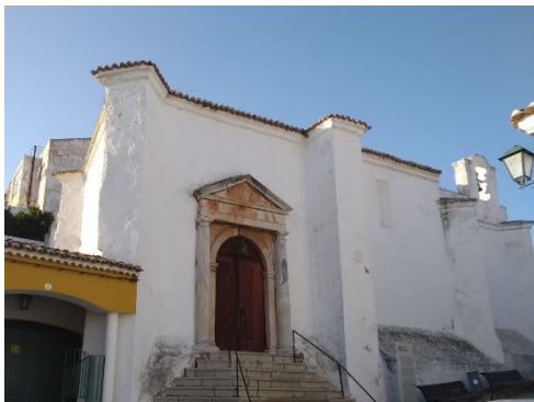
Figure 26 - Structure A: church.
