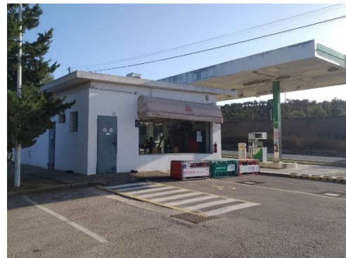
Figure 27 - Structure B: gas station.
