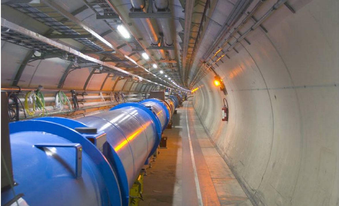
Figure 3.2: View of the LHC tunnel [8]
