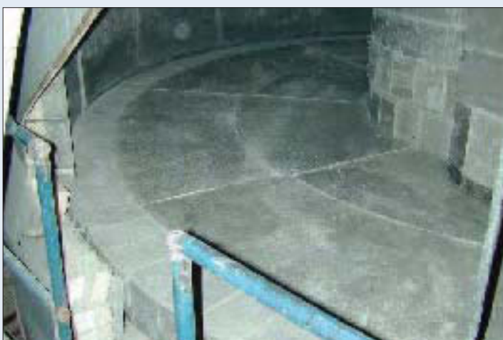
Internal view of the HOTDISC after refractory installation
