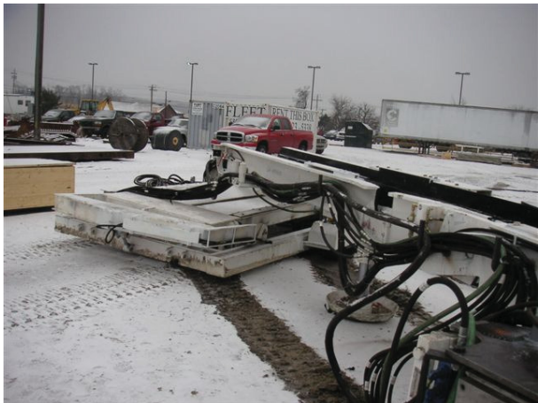
Picture 191: Testing Area outside workshop
