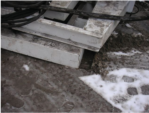
Picture 198: Floor Contact of the Mainframe
