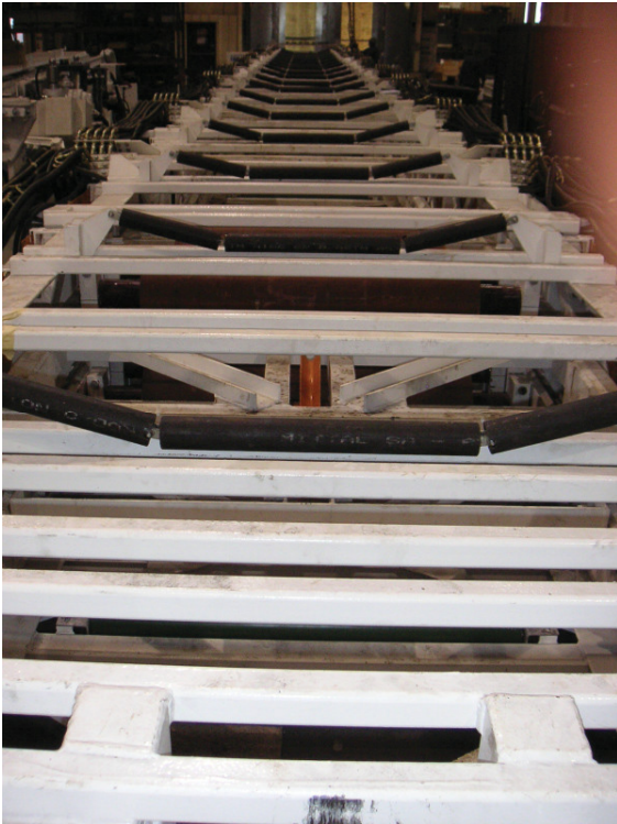
Picture 187: View over top of the LTU unit
