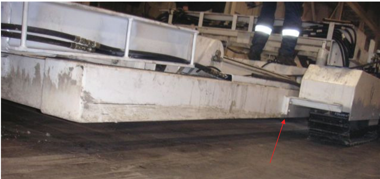
Picture 200: Mainframe lifted 100mm via Track Frames
