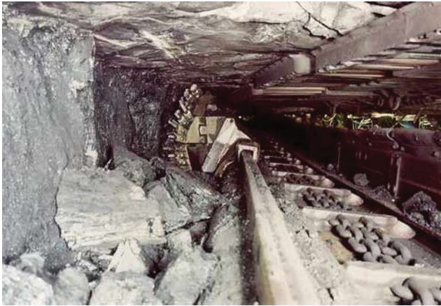
Picture 16: Longwall Plough with Chain Conveyor
