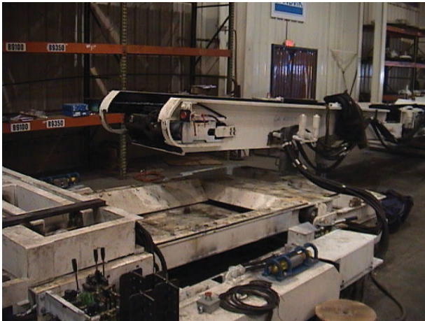
Picture 189: Hydraulic Connections HC and ABM10
