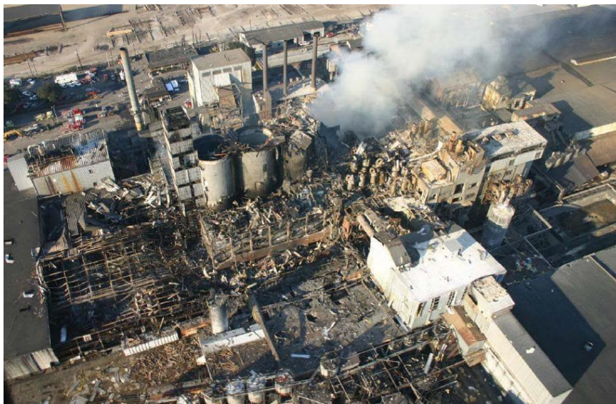
Figure 2: Dust explosion at the Imperial Sugar company on Feb.7 th 2008, Georgia, USA [4]
