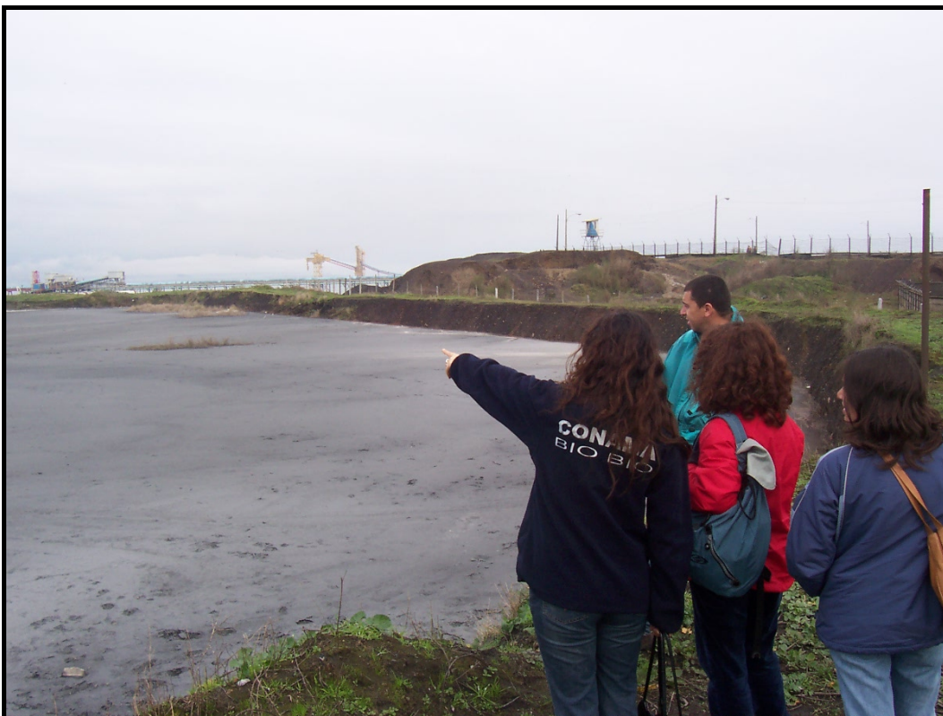
Figure XI.17. Central Bocamina, Coronel.
