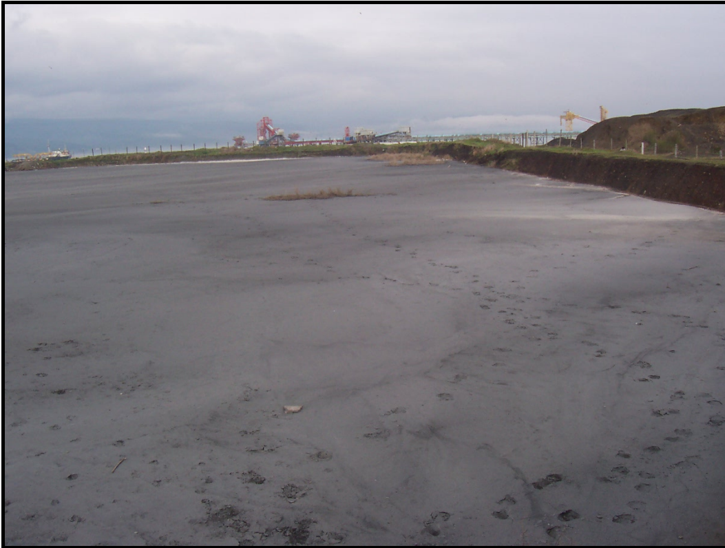
Figure XI.16. Central Bocamina, Coronel.
