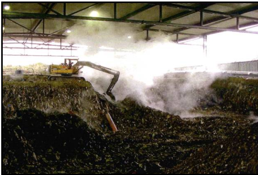
Figure 28. Under roof excavation procedures.
