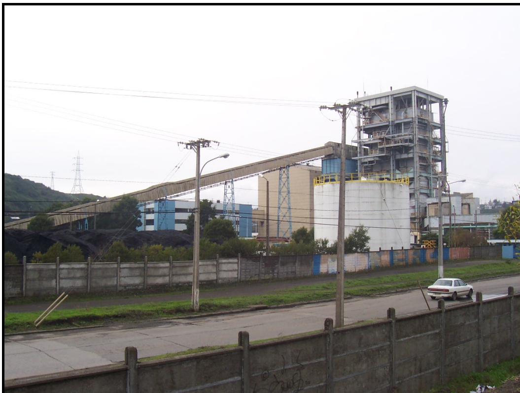
Figure XI.19. Central Bocamina, Coronel.
