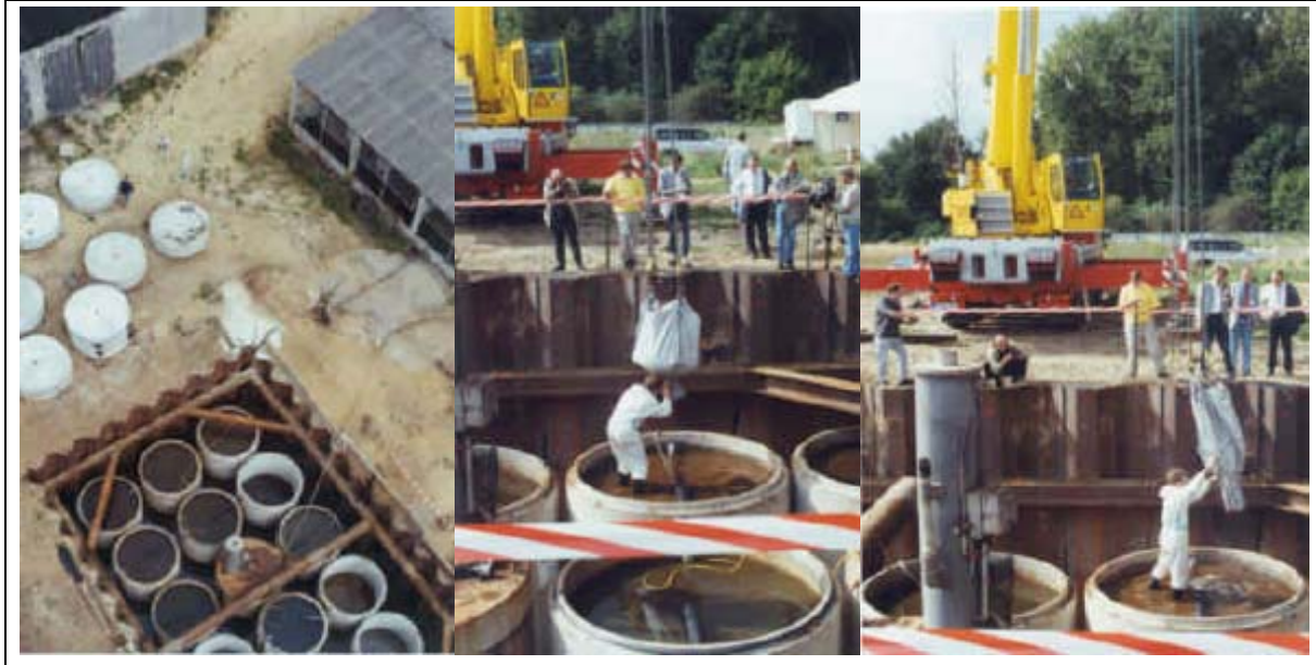
Figure VII-3: Reactive wall reactor modules
