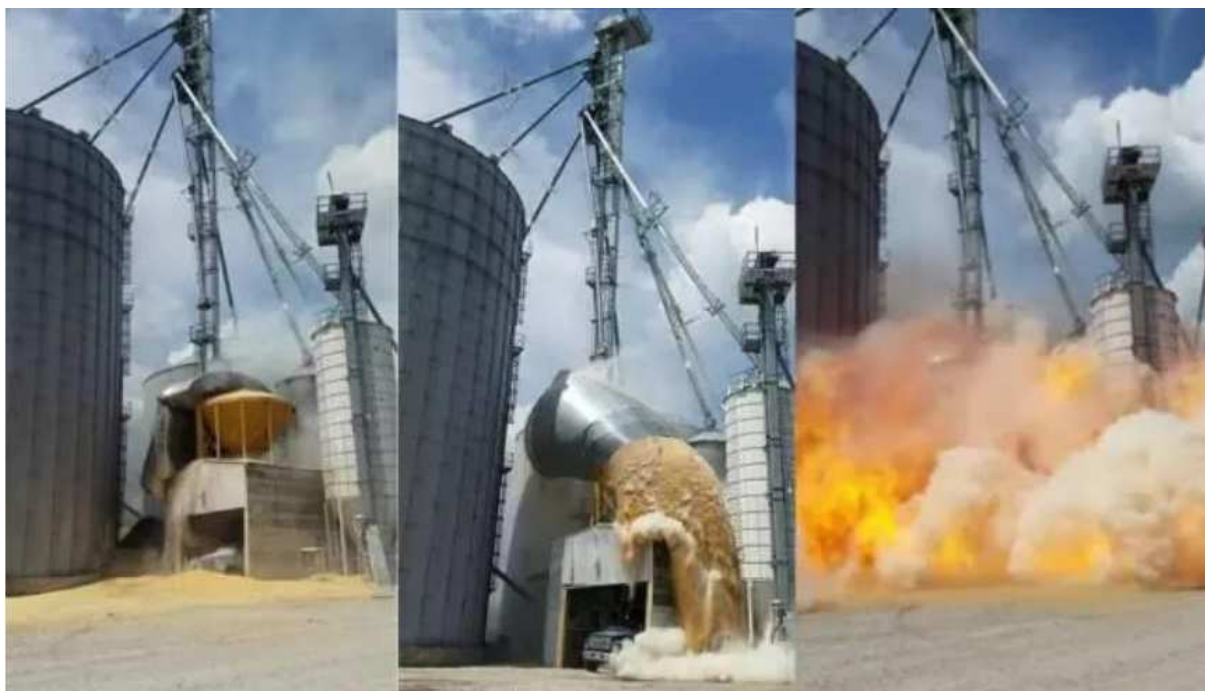
Figure 1.4: An instant of the grain silo explosion in Indiana, USA, 2017 [10].
